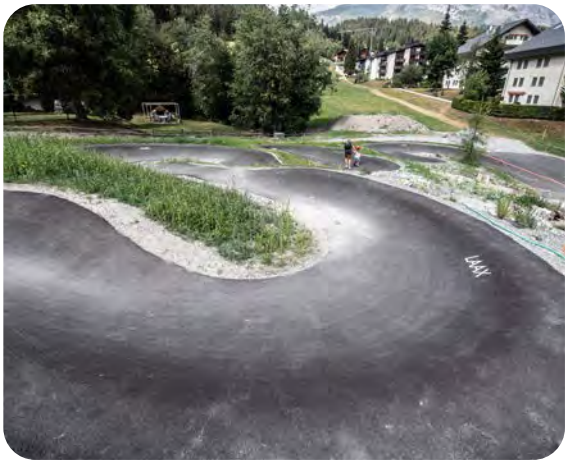
Typical Descending Berm
